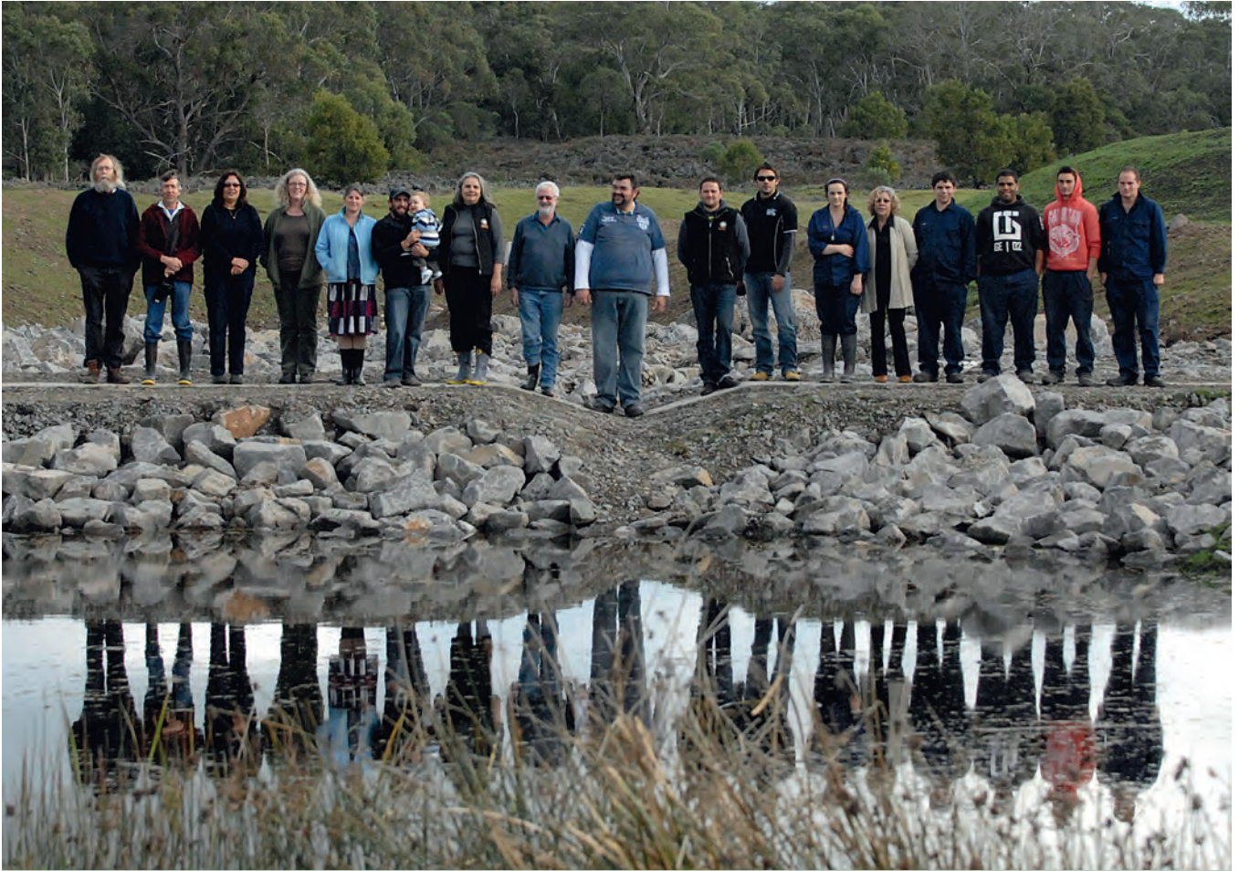
Engineers worked with the indigenous community to build a rock weir that fits in with the surrounding landscape.
